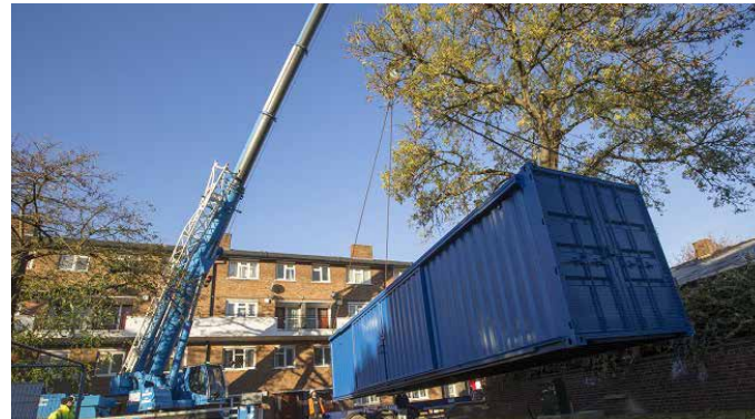
Precedent, Hub on the Solon Estate, Lambeth
